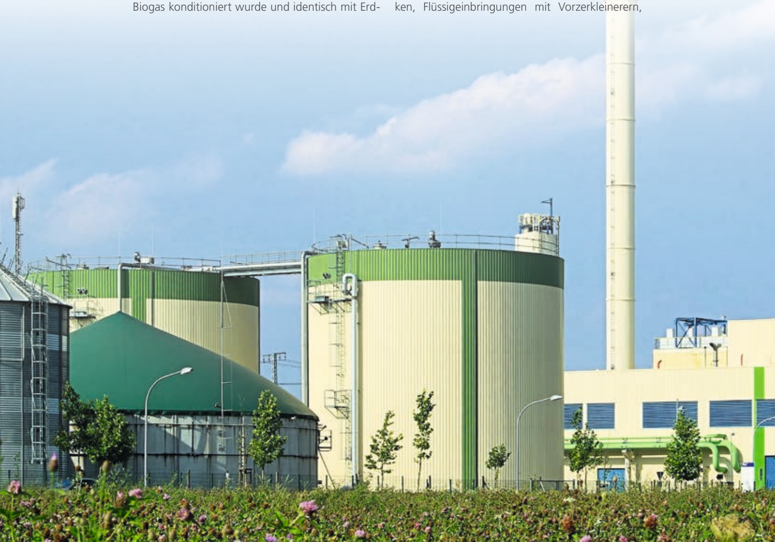
Foto: Biogasanlage - biogas plant 77 © LianeM, fotolia.com / Lagerfotos: Sell Media Company
